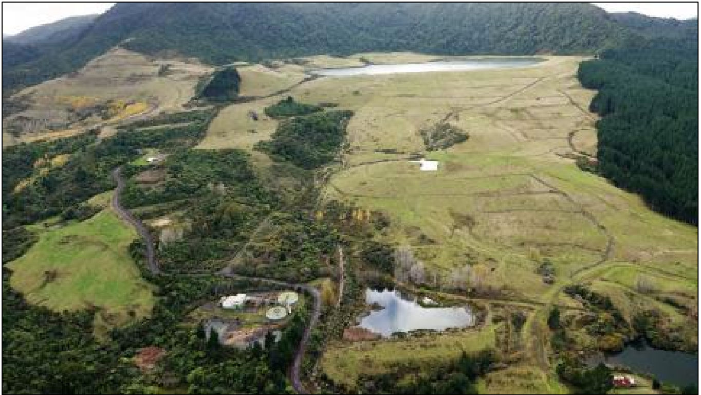
Golden Cross today. The former TSF is visible at the top of the image, close to forested conservation land. The infrastructure at the bottom of the image is the water treatment plant and management system. At the top left, part of the recontoured open pit can be seen.
